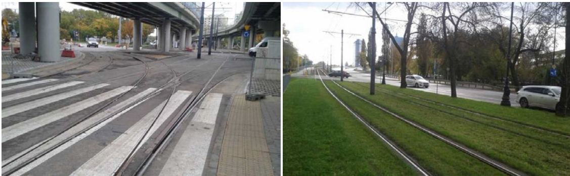
Fig. 1 Integrated on-street tramways and green tramway with used rails 60R2 type.
