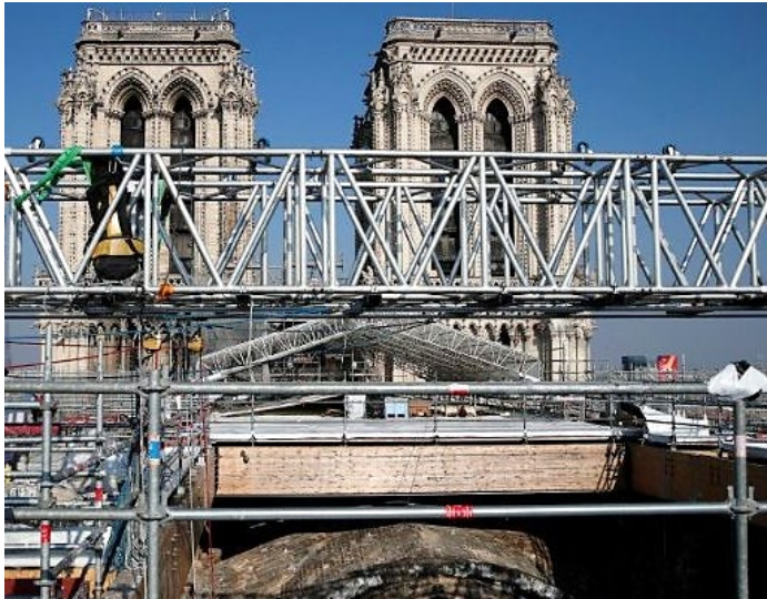
Fig.8. Notre Dame Cathedral, Paris. Restoration work. [17]
