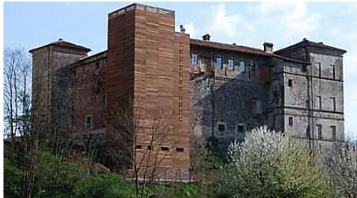
Fig.6. Saliceto Castle, Cuneo, Italy. North-East view, restoration with reconstruction of the tower. [16]
