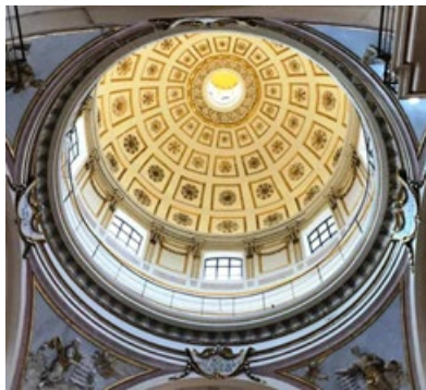
Fig.4. Church of S. Maria del Suffragio, Aquila, Italy- Dome restoration. [12]
