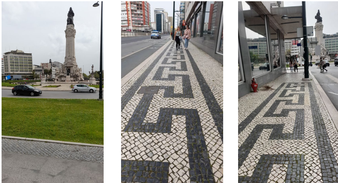
Fig. 1: Center of Lisbon and particular sections of Calçada pavement in Lisbon.
