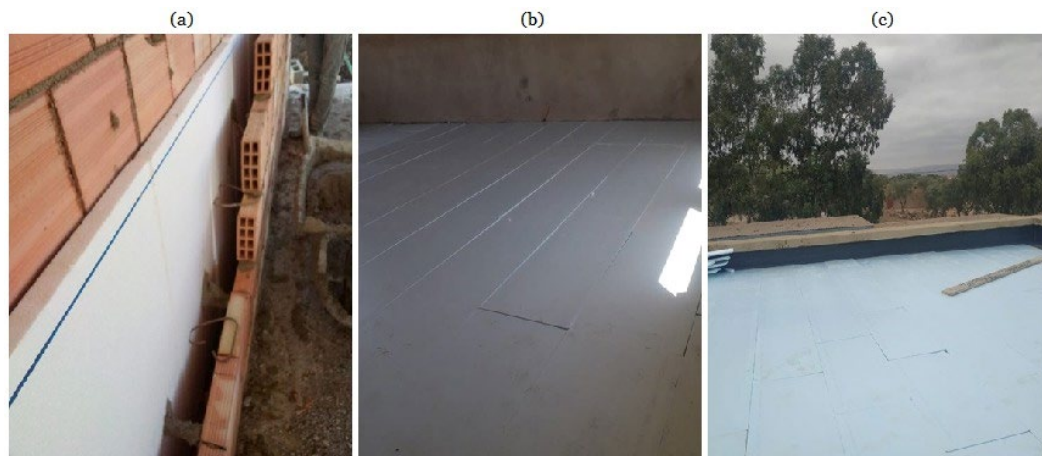
Fig. 6: Installing polystyrene as insulation in the building envelope: (a) external wall, (b) floor on ground, (c) roof.
