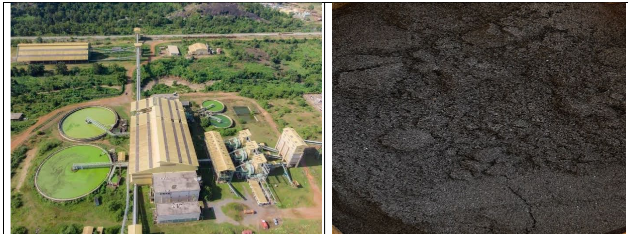
Figure 1: (a) Aerial view of NIOMCO, Itakpe, Nigeria (b) IOT sample
