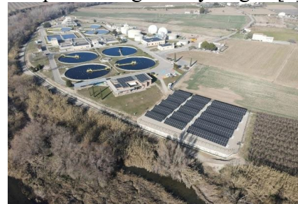
Figure 2. A Water Treatment Facility Operated by Aqualia [2]
