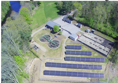
Figure 1. Greenskies 137-kW Solar Array at the Water Treatment Plant [1].
