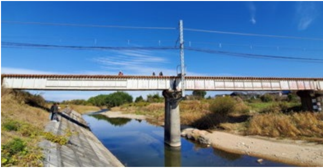
Fig. 1 Monitoring railway bridge pier.
