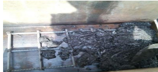
Fig. 2 Photographic View of Casting Reinforced Bendable Concrete Slab
