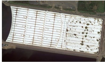
Figure 1. Aerial view of floating cover in western plant treatment
