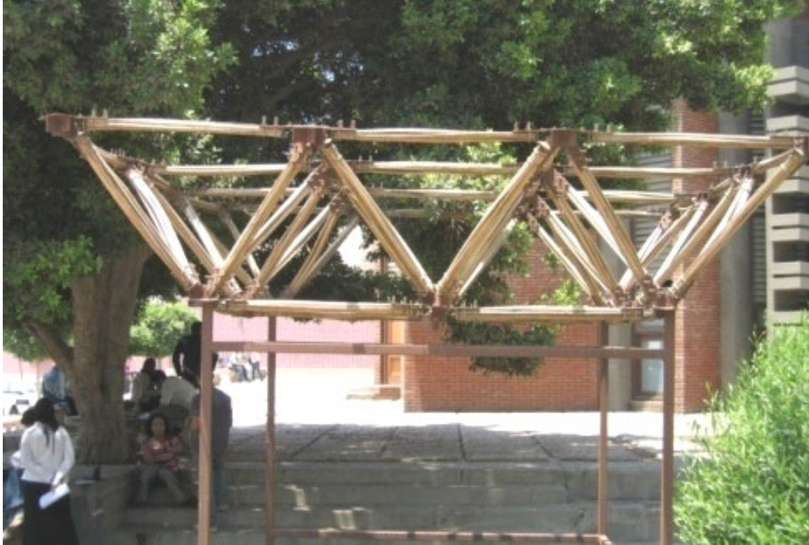
Fig. 20: A prototype of a space truss from palm midribs [16].
