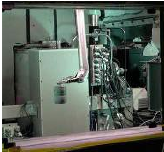
Fig. 8. Quintus HIP unit installed in the HFEF hot-cell at the INL
