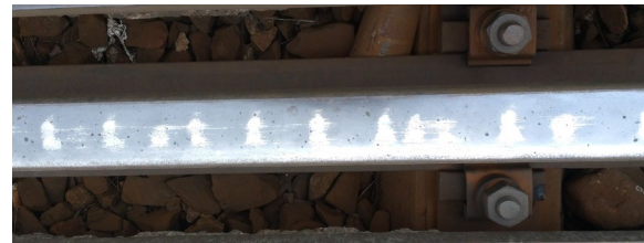
Fig. 2. Defect in rail waviness
